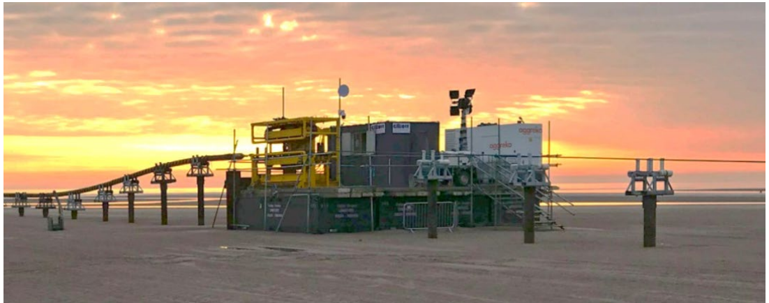
Plate 3.6: Example roller boxes and intermediate pulling platform installation (image courtesy of Boskalis)
